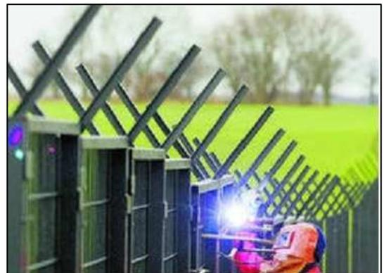
Germany is preparing for the next Group of the Eight meeting. This is the 13 kilometres long, 12.5 Mio. Euro expensive protection fence, which is exclusively built up for the summit. 500 tons of steel, 900 kg cement blocks anchored in the ground, fused bolts, motion detector, video control, microphones.
